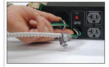
3) Splice conductors together using provided twist-on wire connectors. (factory installed on circuit wiring in the J-Box)
