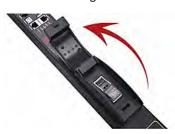
2. Verify the new fuse's rating against the rating specified in the fuse holder's cover.
